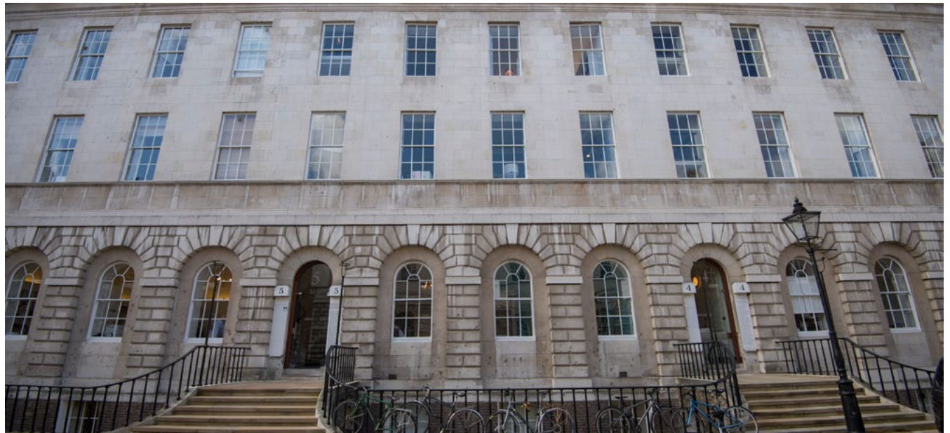
(Lincoln's Inn Stone Buildings)
